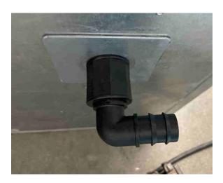
**STEP 8:** Finally, with the cap fastened with the grinder wrench and the reduced sleeve fastened with the parrot beak, we can now tighten the kit so that no water leaks out. It should be screwed until the black piece stops.
