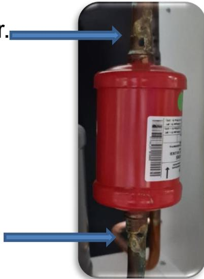
9. Carry out pressurized sweeping with nitrogen through the Refrigeration circuit of the evaporator and suction and liquid pipes.
