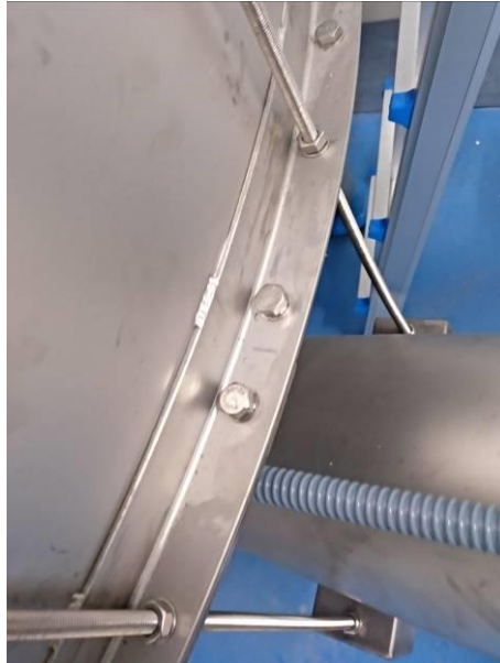
Through holes made so that the flange fastening studs are in line.
