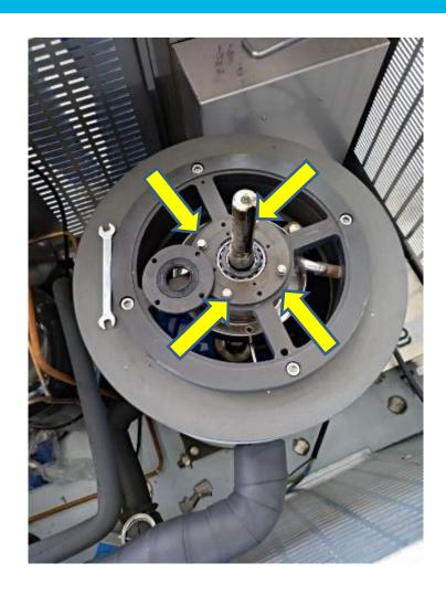
The upper bearing is inside the cover, the 4 screws are removed from the bowl, and it is removed whole (it can be removed together with the upper cross if you do not want to change it)
