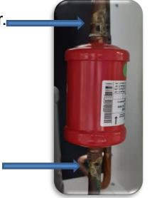
**9.** Carry out pressurized sweeping with nitrogen through the Refrigeration circuit of the evaporator and suction and liquid pipes.
