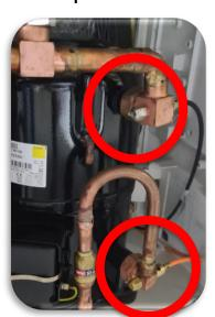
**6.** Remove the oil collector from the compressors
