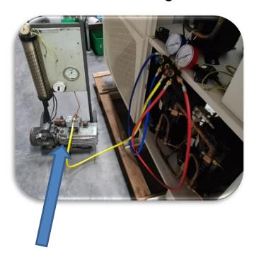
**16.** Once the vacuum has been made, make sure that there are no leaks.
