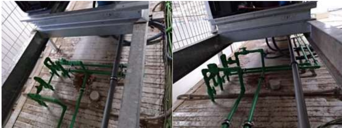
Mounting pipes with bypass in covered shed
